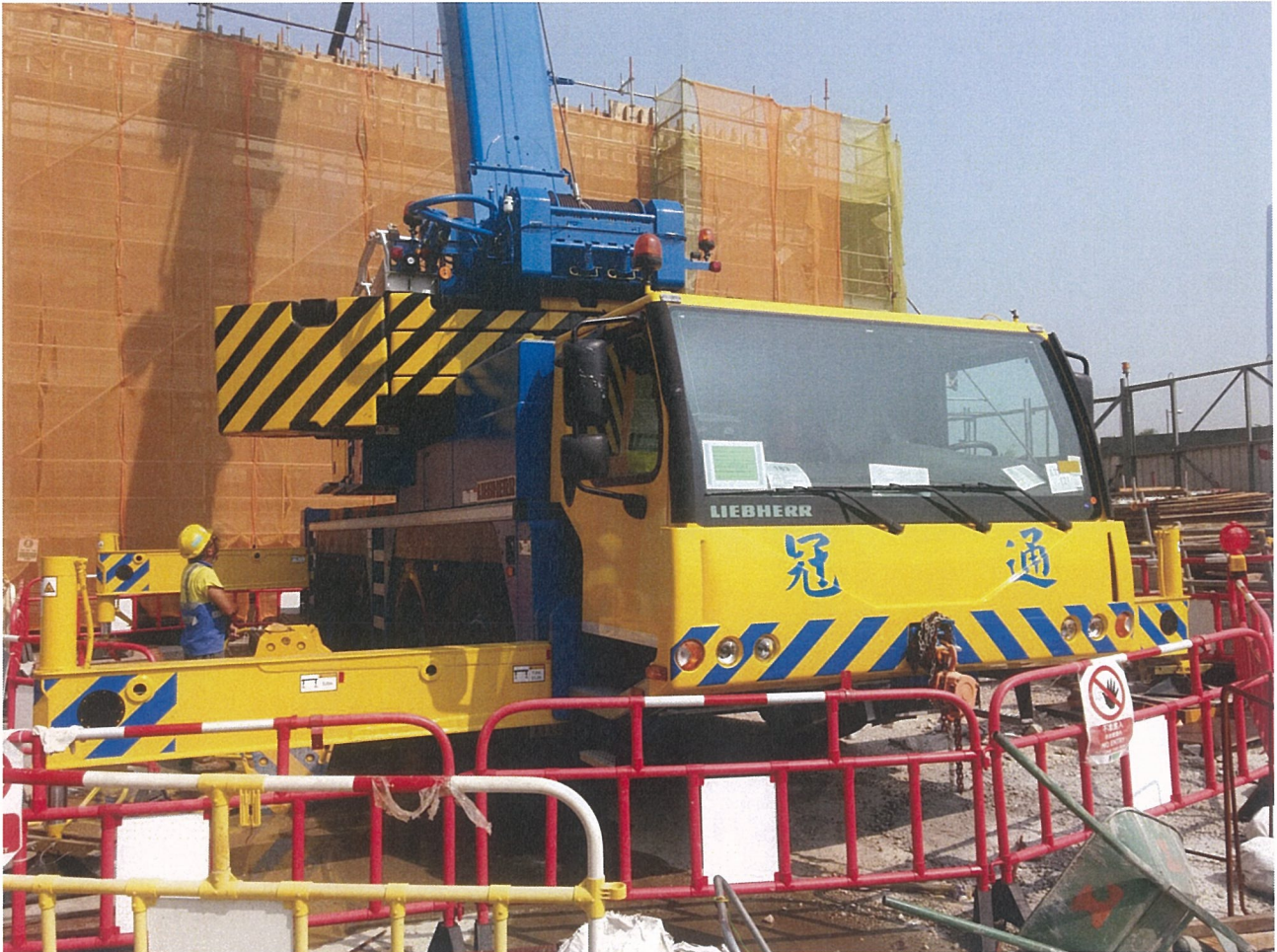
PME Type: Mobile Crane Manufacturer/Model: LIEBHERR LTM 1100-4.2
